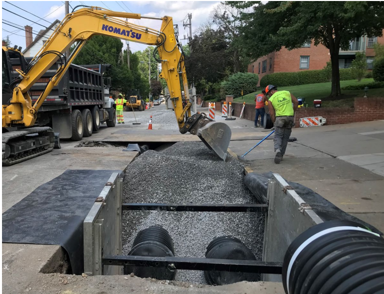
Construction Progress – Stormwater Storage
