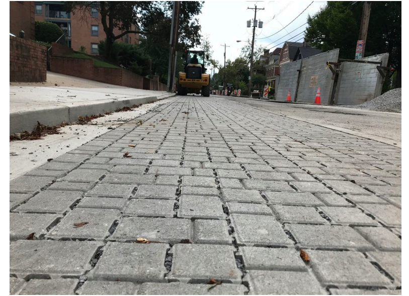
Construction Progress – Completed Pavers Close Up
