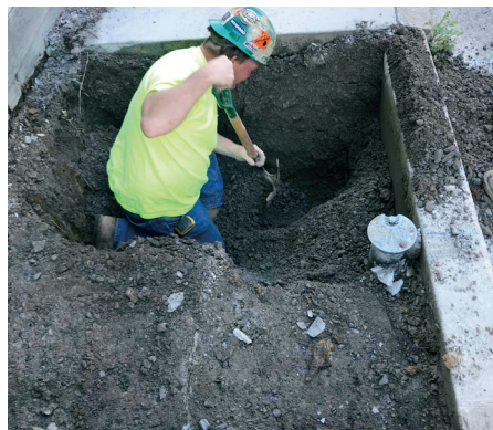
PWSA contractor excavates a lead line in Mount Washington
