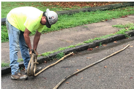
Crews performing lead service line replacement work.
