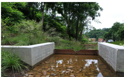
PWSA is building innovative stormwater management systems, such as this one at Centre and Herron. These new systems are designed to absorb, retain, or redirect as much as rainwater as possible before it enters our overburdened sewer system.
