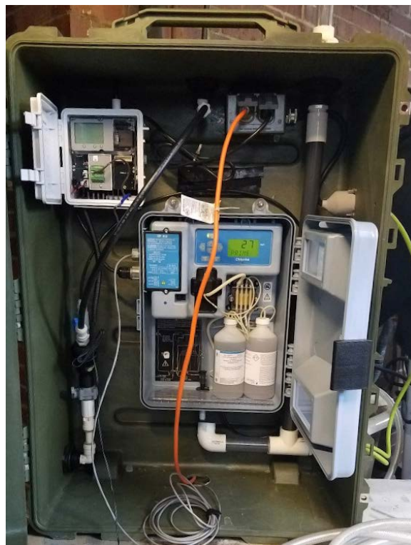
New chlorine monitor installed in the Greenfield Firehouse
