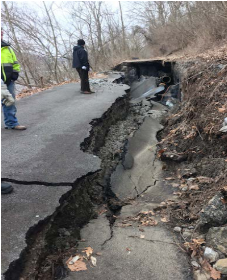
16-inch water main break at the Duck Hollow Trail, February 15, 2019
