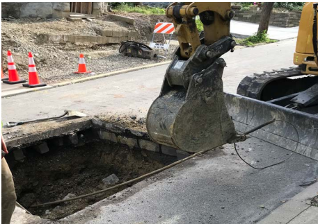
Crews using the “pulling” method, which means PWSA can replace the lead line and avoid digging a trench through the yard.
