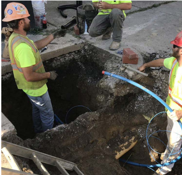
Crews installing a new lead service line
