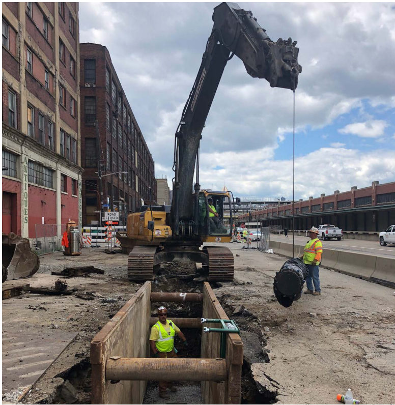
PWSA contractor replacing a water main on Smallman Street
