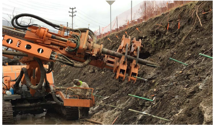
Heavy equipment is needed to drill the soil anchors into the banks of Saw Mill Run.
