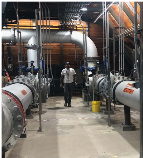
PWSA Production Project Manager, Marc Frangipani, walking through the ultraviolet disinfection chamber.
