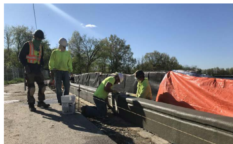
Crews pour concrete wall around Highland Park Reservoir.
