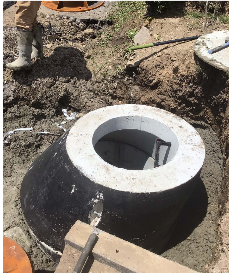
Crews make repairs to a manhole on Keefe Street
