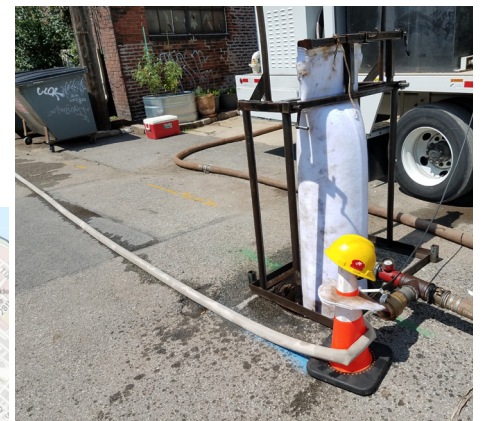
Styrene sewer liner being installed via a manhole.
