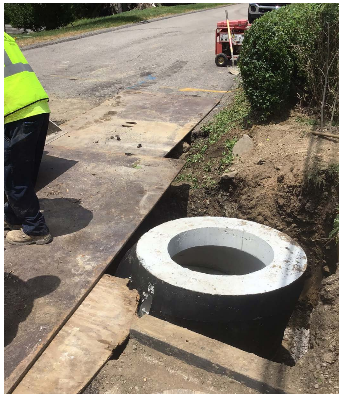
Crews install new sewer manhole on Keefe Street
