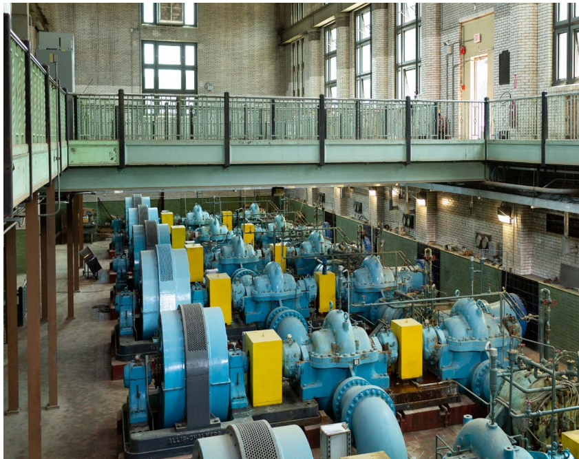
The Bruecken Pump Station was built in 1931. It pumps water from its location along the Allegheny River to either the open Highland I Reservoir or the Highland II Reservoir. From there, water is distributed to customers served by these portions of our drinking water system.
