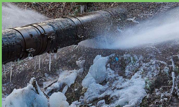
A broken water main prior to being shut off for repair.
