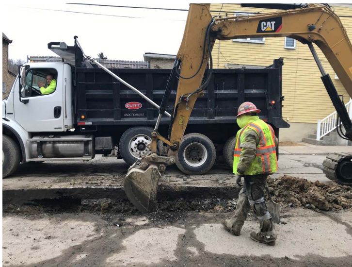
Crews replacing a water main in a Pittsburgh neighborhood.
