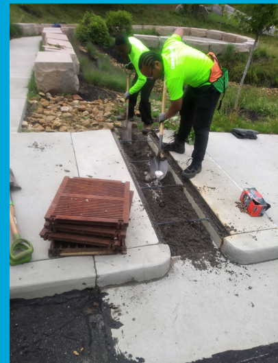
Landforce, a local organization dedicated to land stewardship and workforce development, takes care of the plants and soils for PWSA Green Infrastructure projects by removing debris and weeds so these projects can capture as much stormwater as possible.
