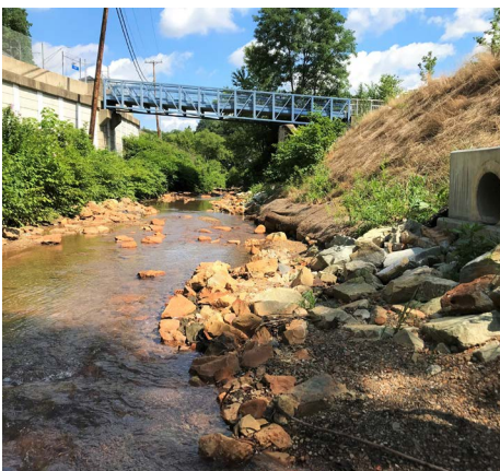
One of three stabilized storm sewer outfalls along the restored Saw Mill Run streambank.
