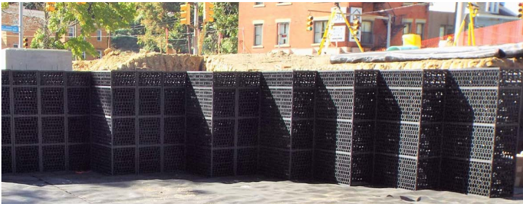
Partially installed R-Tanks at the bottom of the Centre and Herron Stormwater Project in the Hill District.
