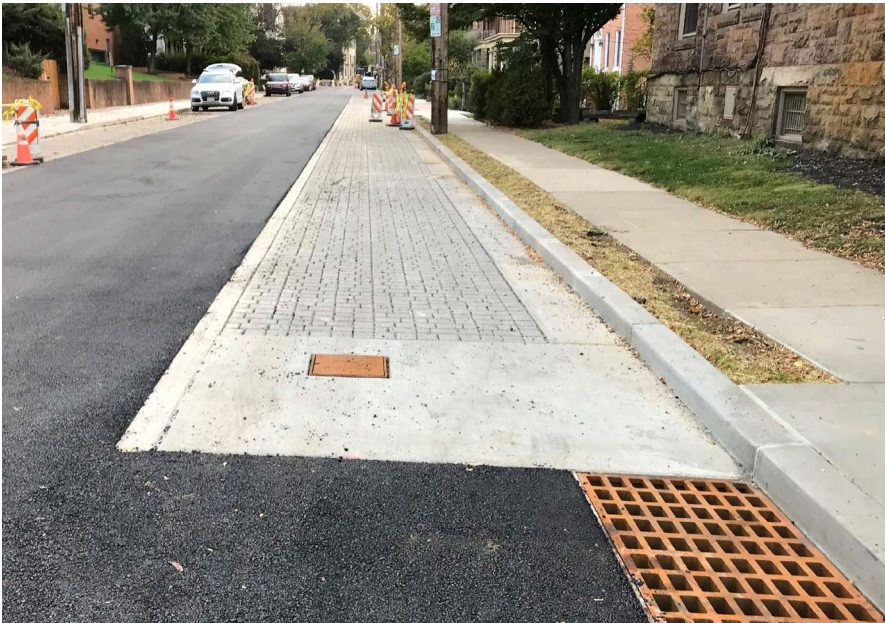
Fresh asphalt and permeable pavers on Kentucky Avenue this fall for the Maryland Avenue Project.
