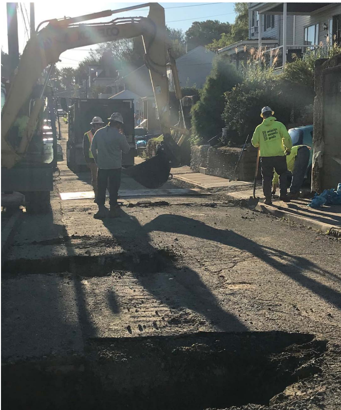
Crews install new service lines during a water main replacement in South Side Slopes.
