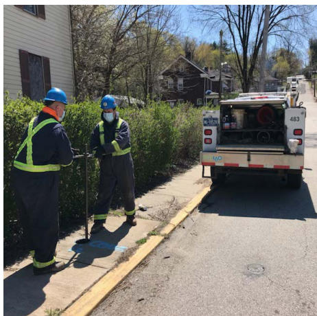
In his role, Joe oversees teams of PWSA Field Operations crews. Above, crews operate a water valve to complete water main repair work.
