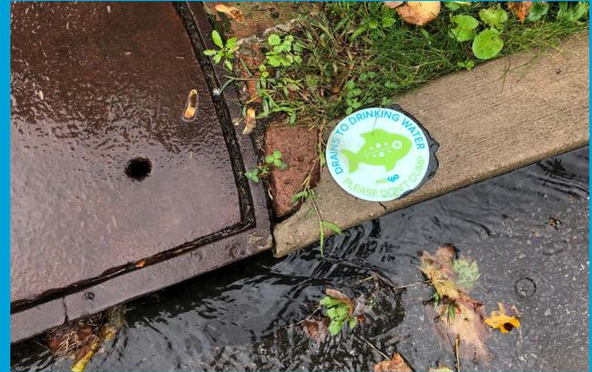
Across approximately 25 percent of Pittsburgh, stormwater and wastewater are routed into separate underground sewer pipes. In these municipal separate storm sewer system (MS4) areas, **primarily located in Pittsburgh's Saw Mill Run neighborhoods**, storm drains on the street carry rainwater directly to our streams and rivers through storm sewer pipes.
