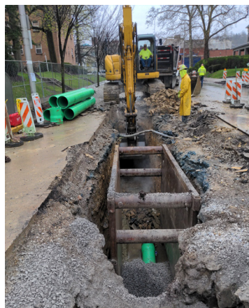
Crews prepare trench for sewer replacement on Centre Avenue
