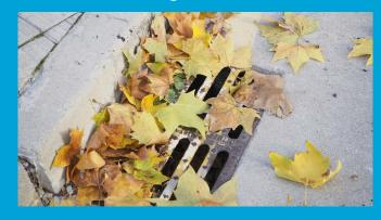
Across approximately 25 percent of Pittsburgh, stormwater and wastewater are routed into separate underground sewer pipes. In these municipal separate storm sewer system (MS4) areas, **primarily located in Pittsburgh's Saw Mill Run neighborhoods**, storm drains on the street carry rainwater directly to our streams and rivers through storm sewer pipes.
