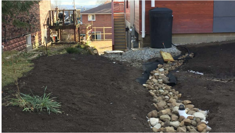
Rich soils surround a rain barrel and serve as an absorbent base for rain garden planting.
