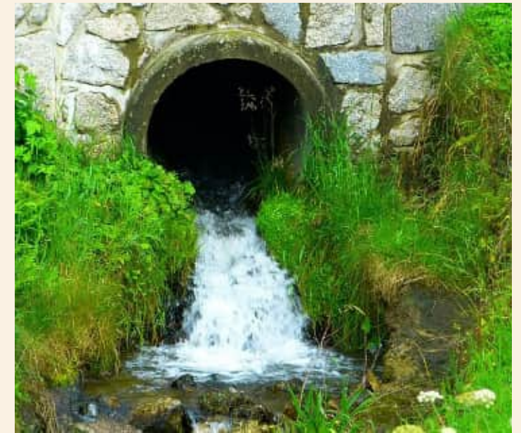
▲ Left: Warning from ALCOSAN that this area periodically experiences sewer overflows. Photo by Meredith Bennett, 2019. Right: Example storm outfall part of an MS4 system
