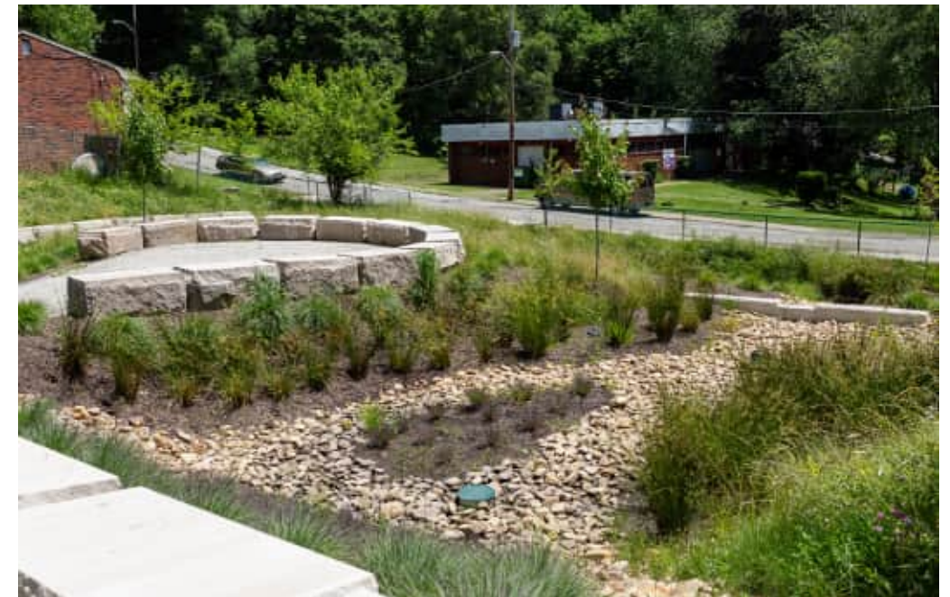
^ Hillcrest Green Stormwater Infrastructure, Pittsburgh
