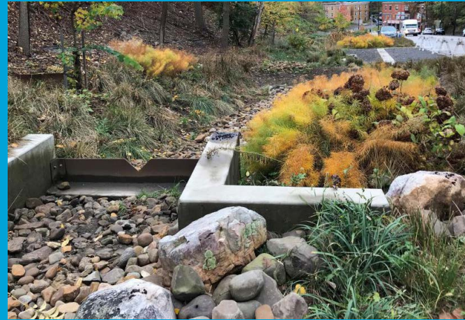
Our Centre and Herron stormwater project in the Hill District.
