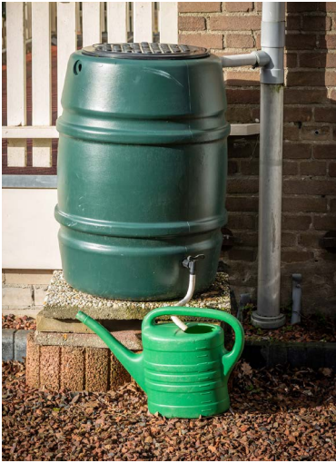
A rain barrel can be connected to your downspout and capture water from your roof for later use. It's a great way to conserve water!
