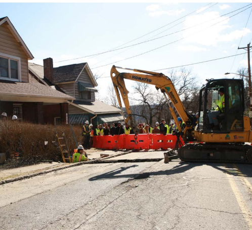
Crews replace the private side of a lead service line.
