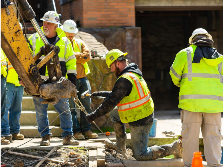
PWSA crews replacing a lead service line.
