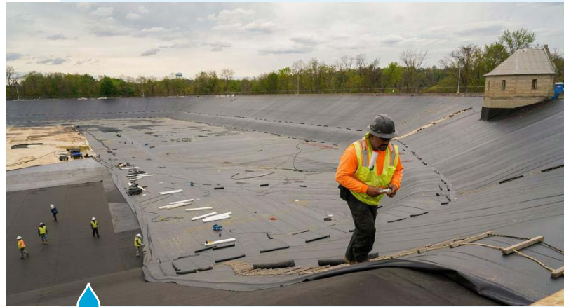
Construction worker adding new liner to the Highland II Reservoir.
